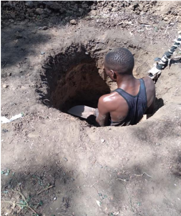
Digging in progress
